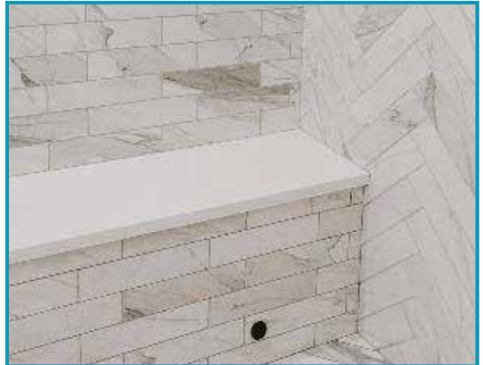
Finished install of nozzles low on wall with nozzle trim.
