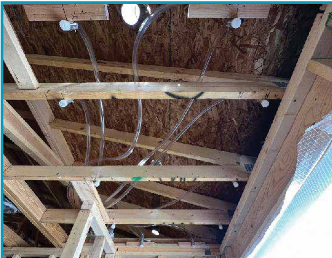
Straight rough in nozzle installed in ceiling to dry down walls.
